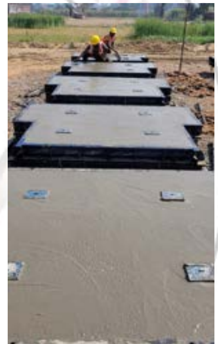
Mould placed on concrete beam.
