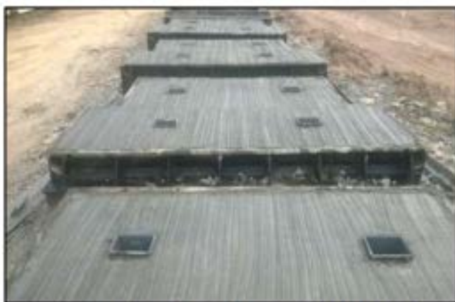
Top surface of panel with broom finish.
