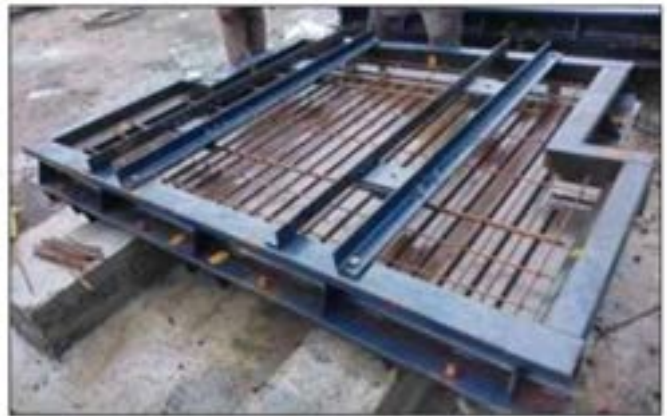
Mould placed on concrete beam.
