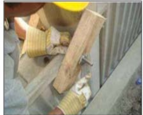
Fixing of clamps between two panels.
